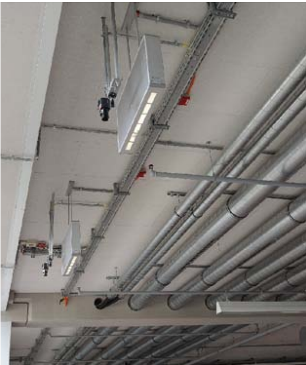
BETA fixss® laying system in use
